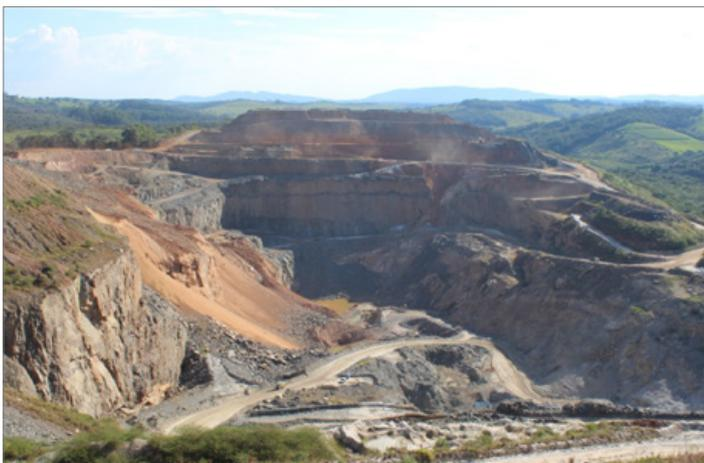
Figure 9: AMG Mineração's Mibra mine in Minas Gerais state, Brazil, contains 20.3 Mt of measured plus indicated resources. Currently it has capacity to produce around 135 t of Ta<sub>2</sub>O<sub>5</sub> per year (photo: T.I.C.)
